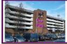
Mitchell Road M15 car park
